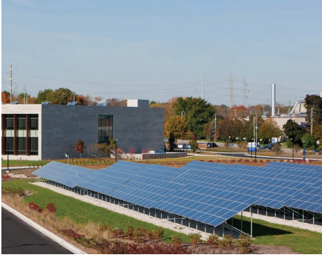
On the grounds, 1,452 solar photovoltaic panels make up one of the largest arrays in Wisconsin, delivering up to 250kW of electricity to the site.
