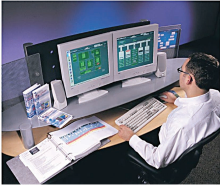
A Metasys® building management system coordinates all control activities across the facilities and provides a single point of access to the information required for optimizing efficiency, comfort and safety.
