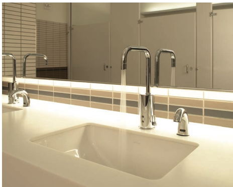
Low flow fixtures and dual-flush toilets significantly reduce water use across the campus. Harvested rain water is used to flush most of the toilets on the campus.
