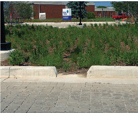
Runoff water is collected through permeable paving on the parking lots and directed to a detention pond, thereby reducing the environmental impact on groundwater and waterways.
