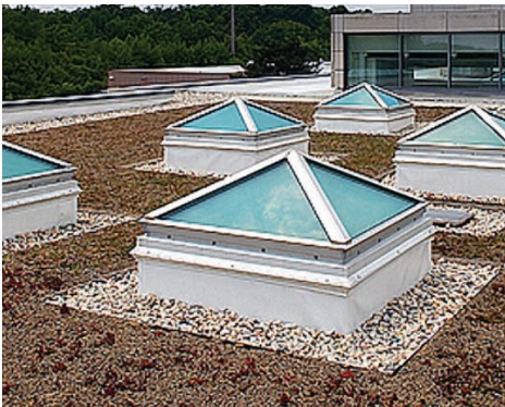
About 12,000 square feet of green roof absorbs precipitation, which reduces runoff, insulates the building, and extends the life of the roof. Skylights reduce the need for lighting inside the buildings.
